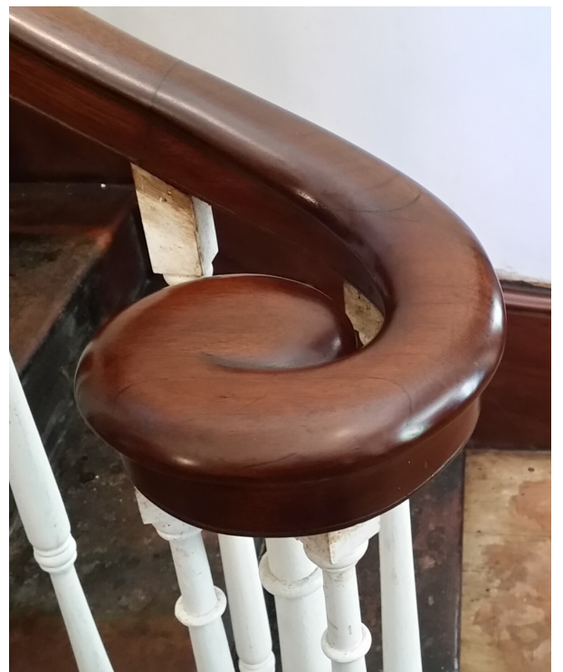
The completed bannister with its new stain and French polish.
