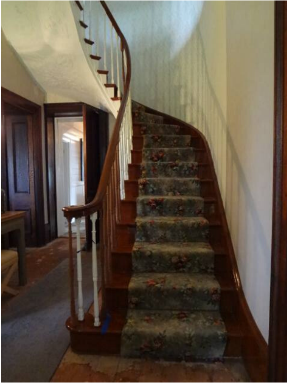
The staircase mid-refurbishment, with the original stair runner and discoloured high-gloss finish. The unpainted balusters are the newly turned ones in cedar.
